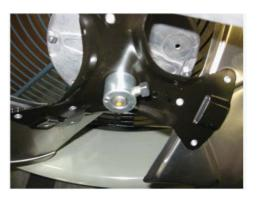
4. Install top assembly to unit using 5/16" screws, and route the conduit through the slot in the control box.
